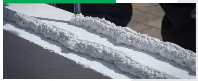
FoamTack Pro Construct is KOMO certified for bonding load-bearing walls. To achieve the best results, we have listed some important guidelines below.
